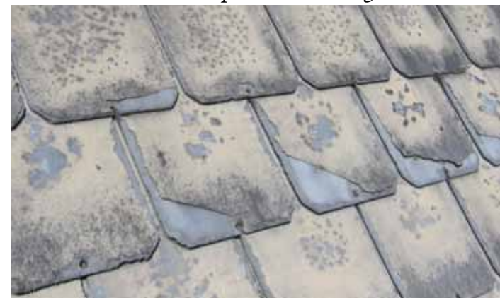
Left: This asphalt shingle roof failed after just seven years. It was reclad using Metrotile Shingle over the existing roof structure. There was no need to remove the original bituminous shingles that were attached to a plywood base.
