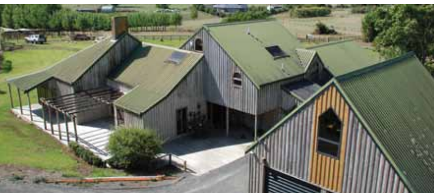
Above: This longrun roof was reclad in Metrotile Shingles as part of a complete "make over" of the original structure.
