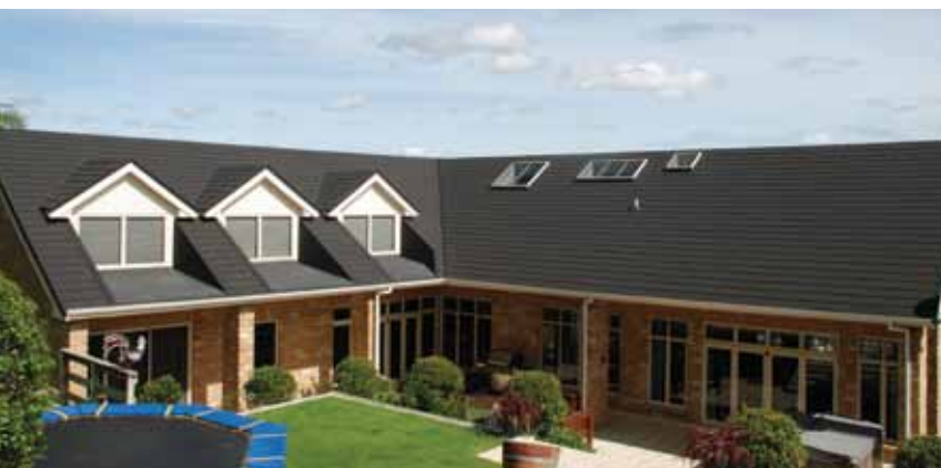
Above: This longrun roof was reclad in Metrotile Shingles as part of a complete "make over" of the original structure.
