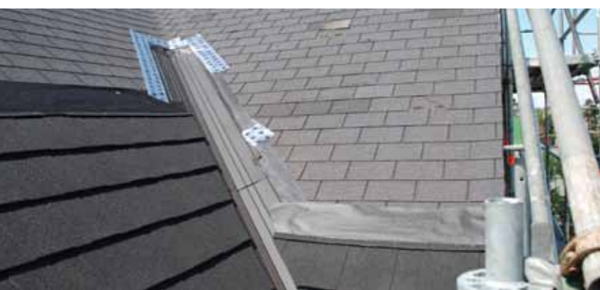
Left: This asphalt shingle roof failed after just seven years. It was reclad using Metrotile Shingle over the existing roof structure. There was no need to remove the original bituminous shingles that were attached to a plywood base.
